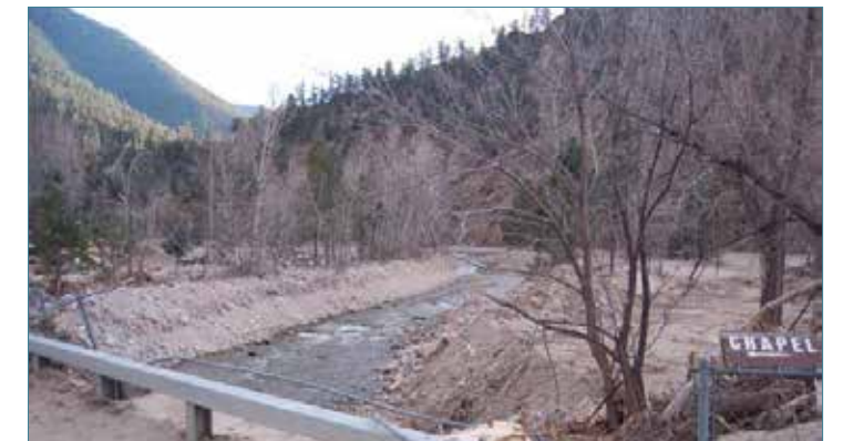
Channelization near Drake. No fish were found at this location post-flood. Source: CPW
